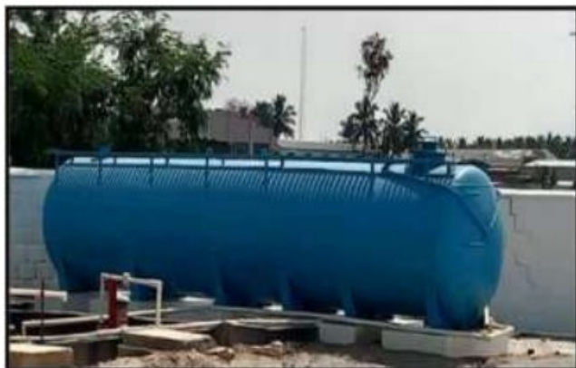
Sulphuric Acid Storage Tank
