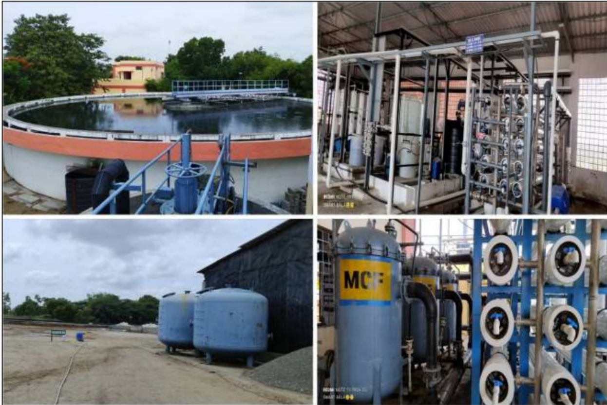
Ultrafiltration, Additional Stage RO and Boilers at Mangalam CETP
