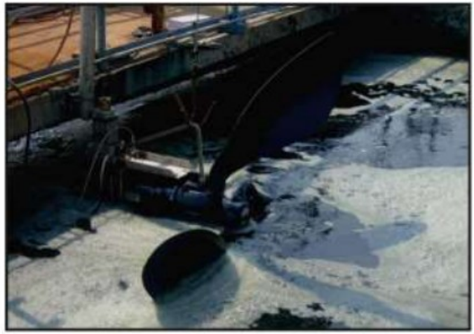
Flow Maker System in BIOT Tank
